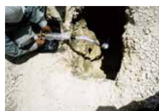
埋設配管 Buried Pipe
